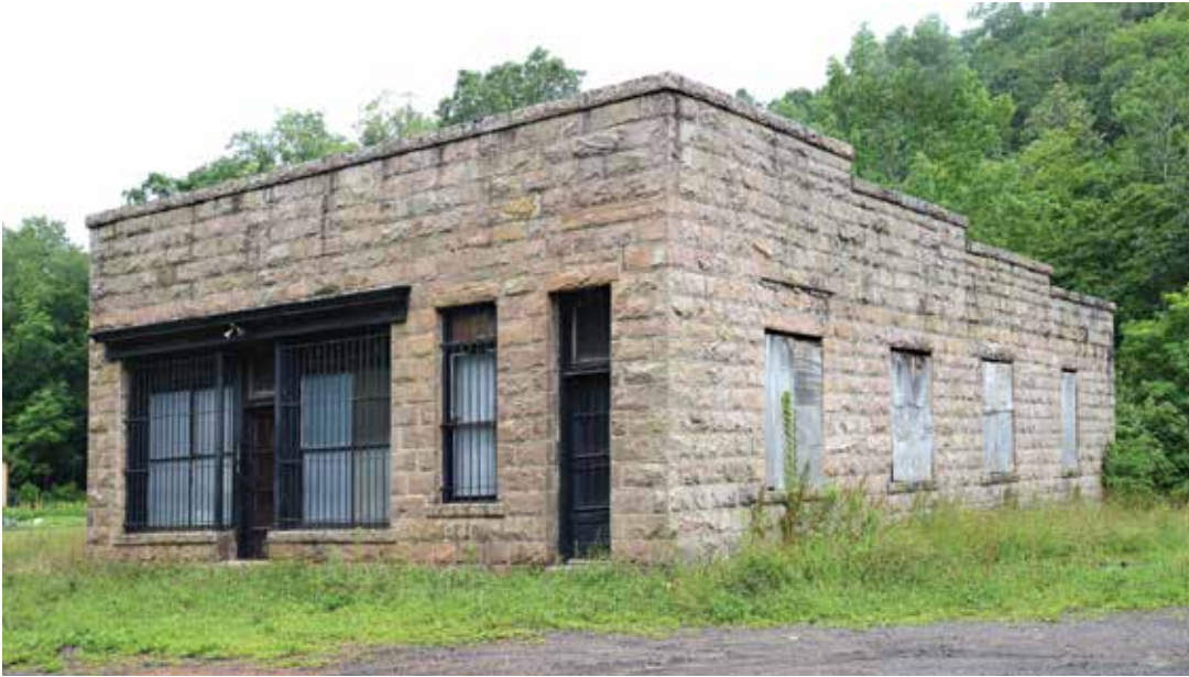
The historical General Store, Post Office, and Wolf Den Coal Company Office was made of local sandstone and cut by Italian stone masons. The building features a tin ceiling, freezers, original counters, and old brass lighting. Built in 1920, this is one of the most historical buildings in Shallmar, Maryland.
