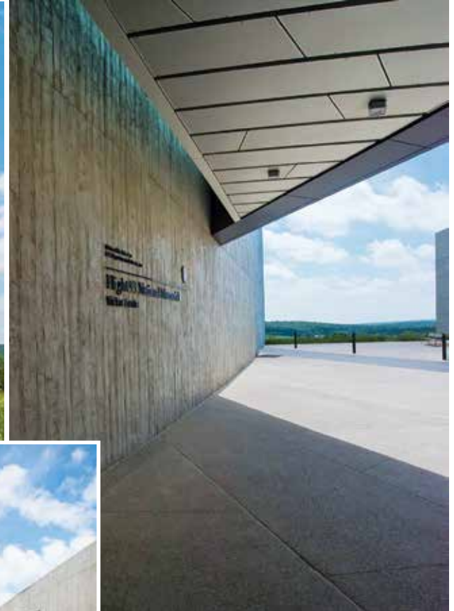
Visitor Center entrance and access to museum and displays.
