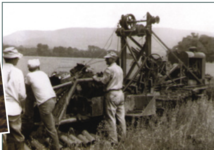
H. Murell Kline (left) and son, William Kline (second from left), work with the owner of the ditch digging machine to lay drain tiles for field drainage in the early 1940s. At that time, their farm had the most fields in the area with a drainage system.
