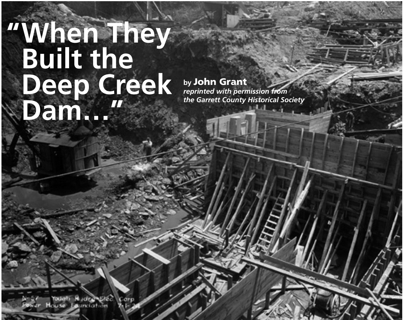
Yough Hydro-Electric Corporation Power House Foundation, July 1, 1924.
