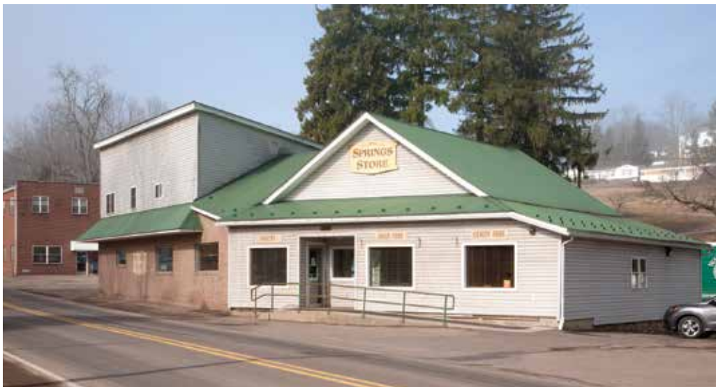
Top: The Springs Store after enclosing the front porch, adding a room for dry goods, and removing the gas pump.
