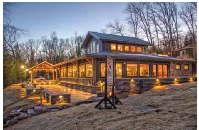
Progression of Firewater Kitchen & Bar from clearing and leveling the property to final building.
