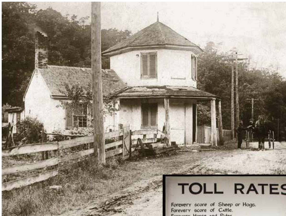
The LaVale Toll Gate House, 1907 1907 GILBERT PHOTO STUDIO, COURTESY ALBERT AND ANGELA FELDSTEIN
