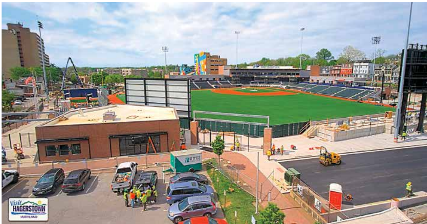
Construction progress at press-time (May 1, 2024). Opening day is scheduled for May 17, 2024.
